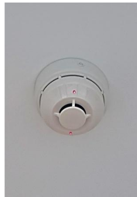
Apartment smoke detector with alarm LED illuminated
